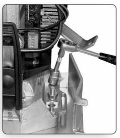
Tighten nuts progressively i.e. left hand, then right hand, then left hand. Do not over tighten nuts.
